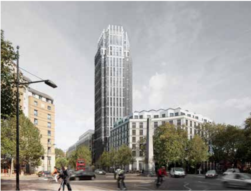
Above Blackfriars Circus, in Southwark, by Maccreanor Lavington for Barratt Homes. Status: under construction
