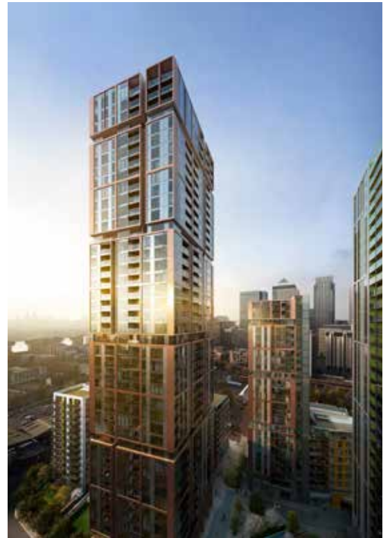
Right Harbour Central, in Millharbour, Tower Hamlets, by Rolfe Judd for Galliard Homes Limited. Status: under construction
